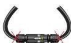
Incorrect Routing of cable
