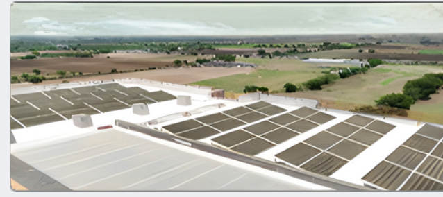
Marwadi Group upcoming 1.7MW Project in Chotila Rajkot.
